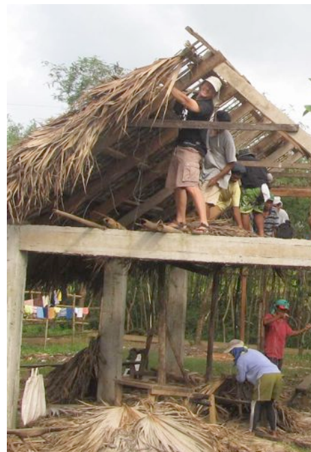
Standing on the beam (this time cement) & installing another leaf in our new Maliktay, San Miguel Island Chapel (Our former chapel will be used for Sunday School)
